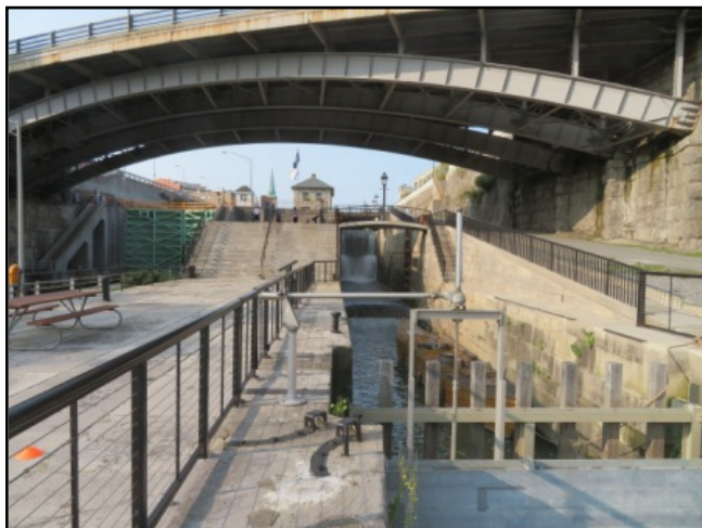
Figure 7. Flight of Five at Lockport on right, original steps center, and the New York State Barge System locks at left.
